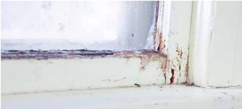
Replacement of windows with lead-based paint hazards (above) with new energy efficient windows (below) reduces exposure to lead contaminated dust and prevents lead poisoning.
